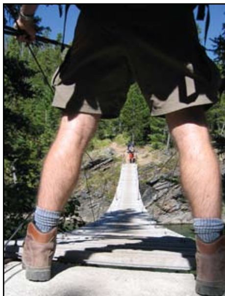
Waterton River Bridge - photo by Brian McKeon
