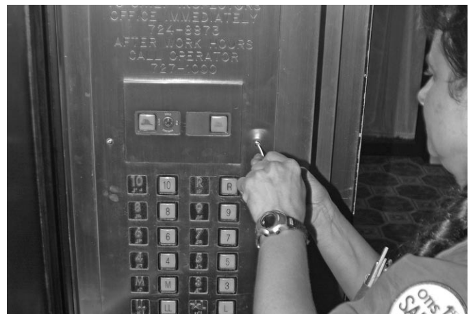
Repairers make sure that an elevator operates according to specifications and stops at each floor within a specified time.
