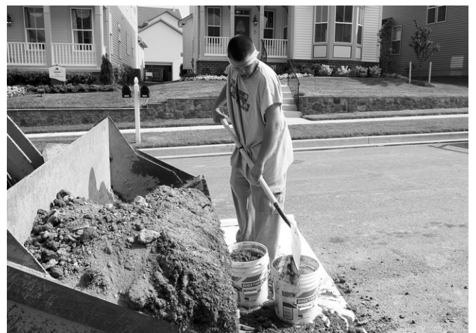
Construction laborers remove excess materials after a job is completed.
