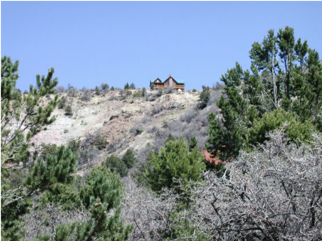
Home threatened by a small landslide that has formed on the headwall scarp of the much larger Green Hollow landslide near Cedar City, Utah.
