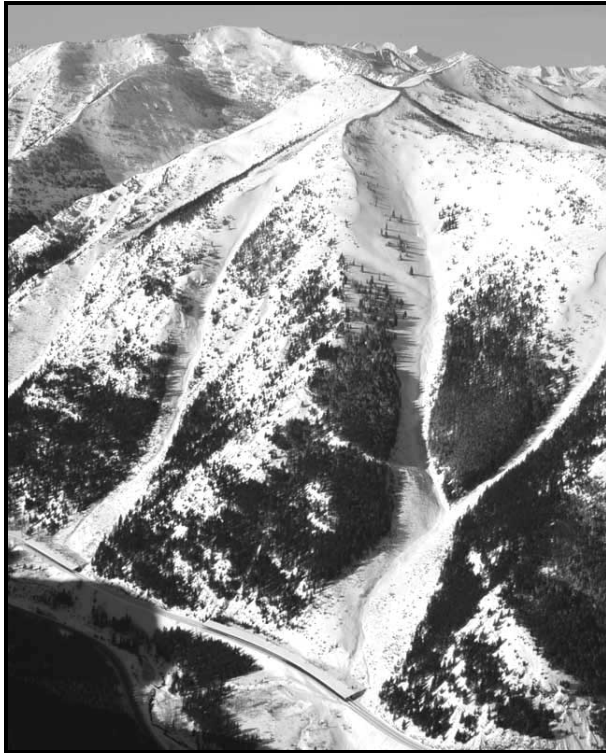
Figure 5: Aerial photo showing (L-R) Shed 8 and Shed 7 avalanche paths on Snowslip Mountain, with cornices formed by prevailing west winds. Visible in lower center is east end of Shed 7, where slides have blocked entrance to the shed numerous times. Photo by D. Stoneman.
