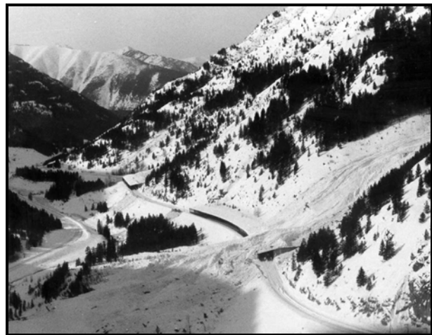
Figure 11: Photo looking west down John F. Stevens Canyon at debris over Shed 7 and Shed 8. Highway on left. Photo Feb. 15, 1979 by M. Martinelli.
