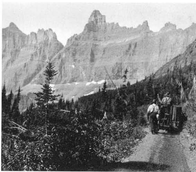
FIGURE 1. Oiling of backcountry trails to eliminate the “dust menace,” circa 1932. Glacier National Park management and archive documents indicate that certain trails were oiled from valley-bottom up to alpine passes.
