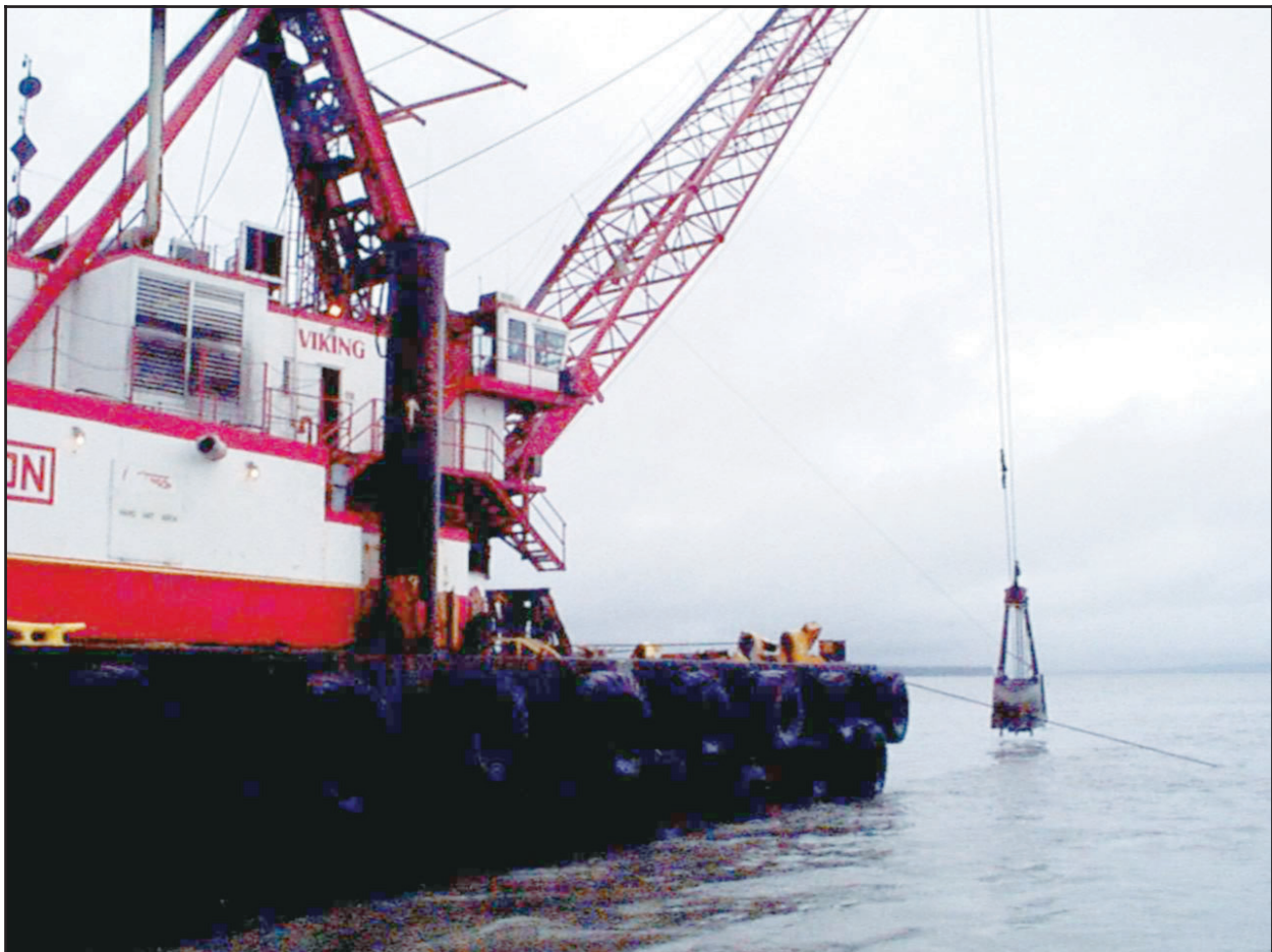
Figure 2. Bucket dredge Viking operating in Cook Inlet, Alaska
