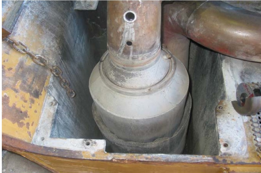
Figure 6.—DCL MINE-X Sootfilter DPF system on haul truck #99942.
