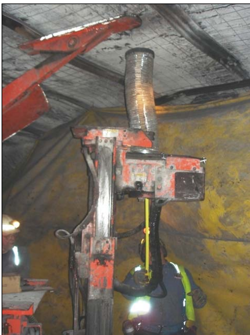
Figure 3.—As drilling advances, the CDSE collapses.
