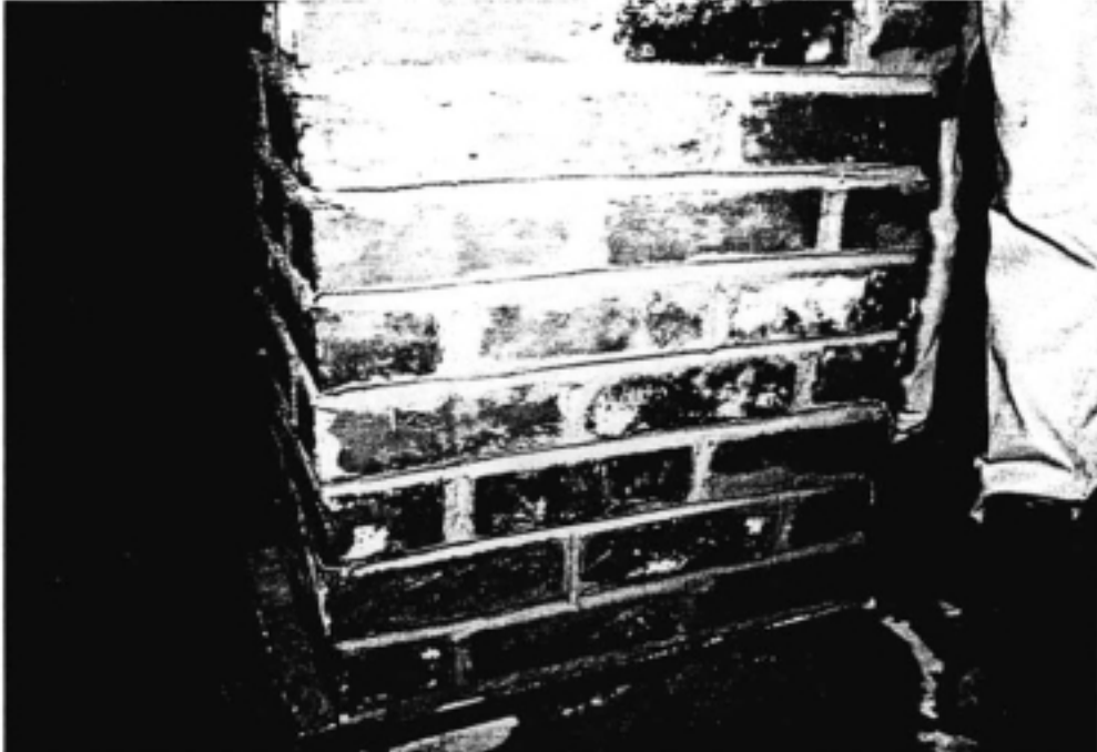
Figure 4.4. The tooled joints of a pier.
