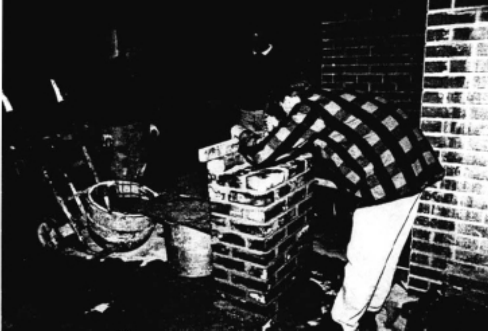
Figure 4.2. Checking for horizontal level during pier construction.
