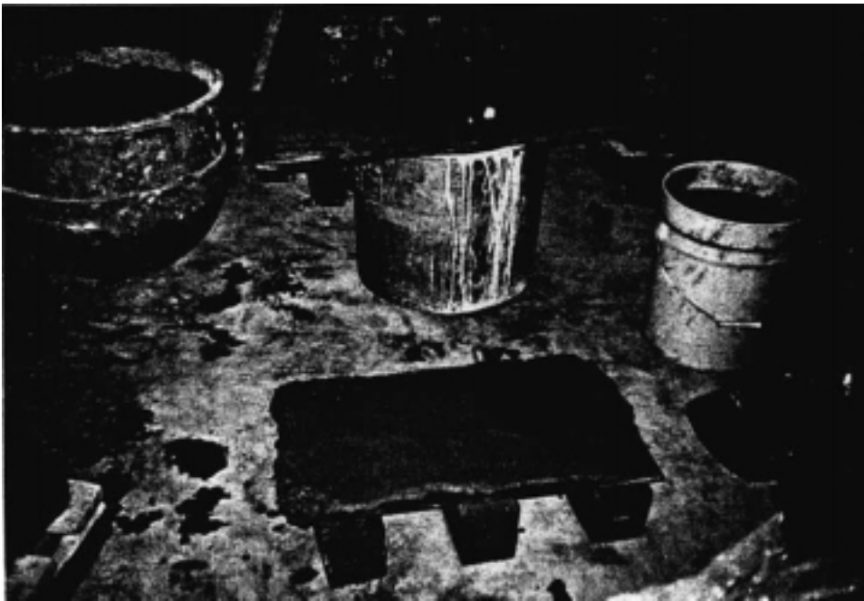
Figure 4.1. Steel plate with mortar base prepared for pier construction.
