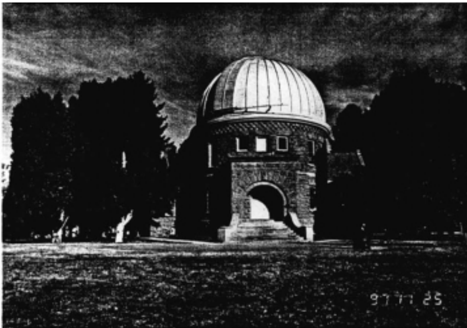
Figure 7.4. South elevation of the Chamberlin Observatory.
