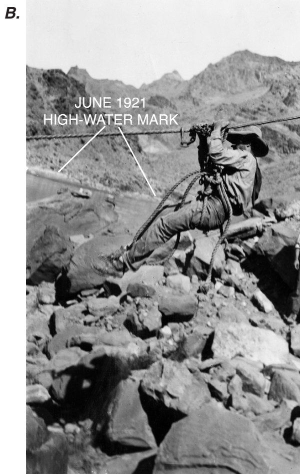
Figure B1. Repairs to the Upper Cableway and the high-water marks from the 1921 flood (photographs by R.C. Rice, U.S. Geological Survey, September 20, 1921). (A) View from the right bank of the cable and cable car in the river in the morning. High-water marks from the June 1921 flood are visible on the left bank. Source of this and the photographs in figs. B1B–B3D, and B4–B6: 1921–37 Surface Water Records File, Colorado River at Lees Ferry, Arizona, file stored at the Federal Records Center in Laguna Niguel, California, in Accession No. 57-78-0006, Box 2 of 2, Location No. MB053635. (B) Downstream view from the right bank of Sid Wilson attaching the chain come-along to the cable. High-water marks from the June 1921 flood are visible on the left bank in the background.
