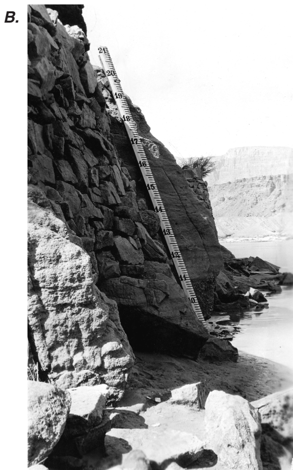
Figure B2. The Dugway Gage and the high-water mark from the 1921 flood (photographs by R.C. Rice, U.S. Geological Survey, September 22, 1921). (A) Downstream view of the vertical low-water section (on right) and inclined middle section (on left) of the Dugway Gage. (B) Downstream view of the inclined middle section of Dugway Gage.
