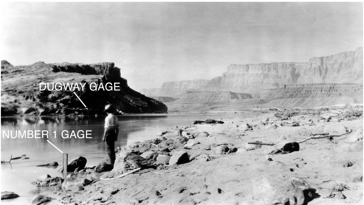
Figure B4. The Number 1 Gage (photographs by R.C. Rice, U.S. Geological Survey, September–October 1921). (A) Downstream view of the inclined higher-water section of the Number 1 Gage on about September 20, 1921. This was the gage built by the observer, Frank T. Johnson, after the crest of the June 1921 flood. It was read by taping down from a nail used as a reference point. The trench was dug to connect the gage to the river. The vertical low-water enamel section had not yet been installed when this picture was taken. Peak stage of the June 1921 flood was measured at 30.89 feet on this gage. This stage equals an elevation of 3,133.50 feet above the NGVD1929. (B) October 3, 1921, downstream view of the vertical low-water section of Number 1 Gage installed by Roger C. Rice on September 25, 1921. Elmer Johnson, assistant gage observer and hydrographer, standing next to gage. Location of Dugway Gage on the left bank is indicated.
