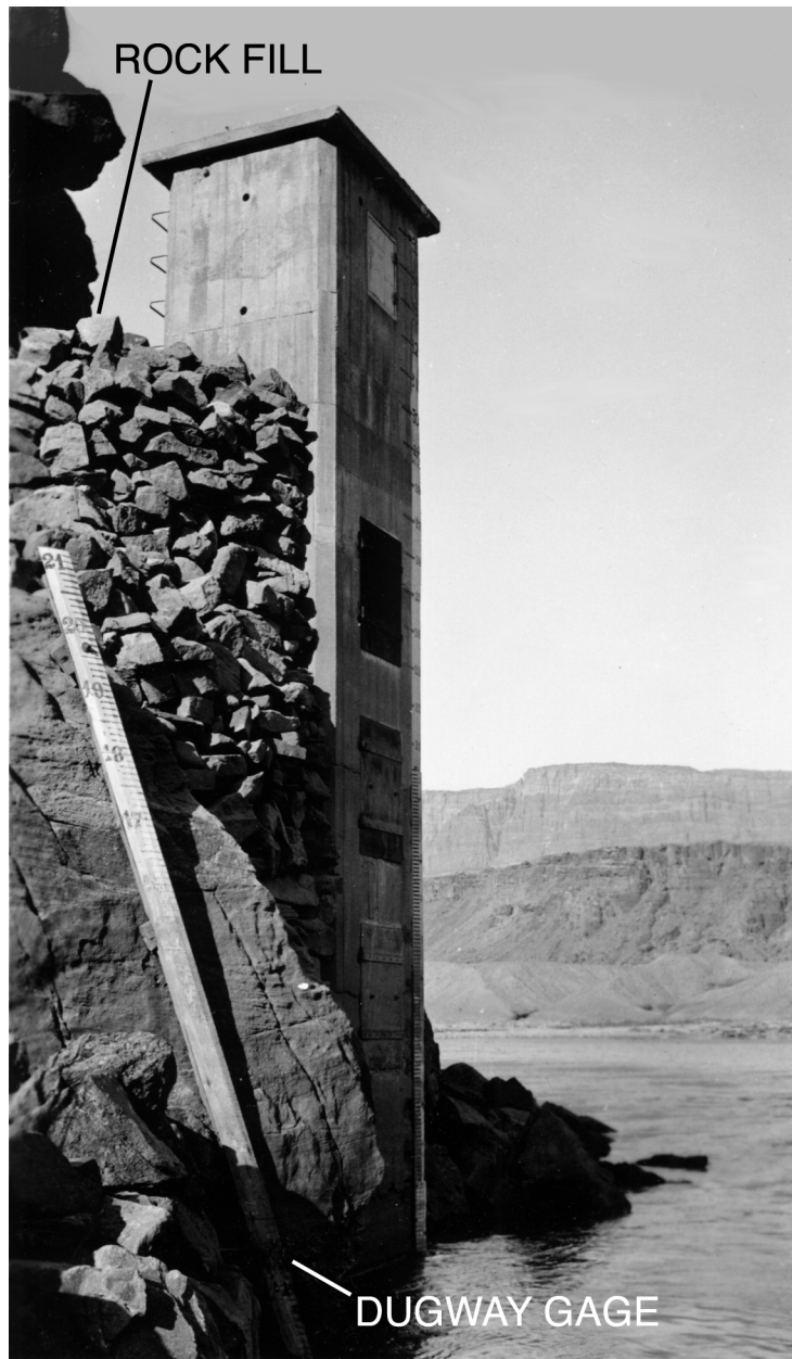
Figure B6. March 1933 downstream view of the Lees Ferry Gage and the high level of the rock fill placed behind the gage in 1929–30. The inclined middle section of the old Dugway Gage is in the foreground; compare to view in fig. B2B. (Photo taken by the U.S. Geological Survey.)
