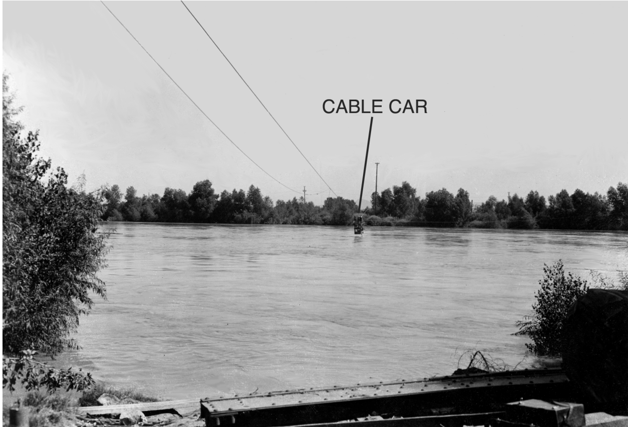
Figure 10. Discharge measurement being made by the U.S. Reclamation Service (the former name of the Bureau of Reclamation) on the morning of June 27, 1921, at the Yuma gaging station, near the peak of the June 1921 flood. At the time of the photograph, measured discharge (based on the measured surface velocity and a coefficient of 0.9) was 182,000 cubic feet per second, and stage was 31 feet. Photo "Yuma 1094" taken by the U.S. Bureau of Reclamation. Source of this photograph: 1891–1937 Surface Water Records File, Colorado River at Yuma, Laguna Niguel Federal Records Center, Accession No. 57-78-0006, Box 2 of 2, Location No. MB053635.
