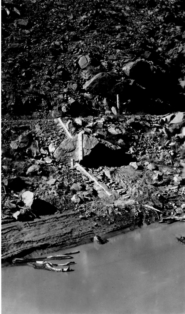
Figure B3—Continued. The Number 4 Gage and the high-waters mark from the 1921 flood. (D) October 2, 1921, view of the inclined upper sections of the Number 4 Gage. Analysis of figs. B1D, 3A, and 3B indicates that the peak stage of the June 1921 flood was at about the elevation of the road in this photograph. This elevation equals a stage of 27 feet on the Number 4 Gage, which equals an elevation of 3,133.9 feet above the NGVD1929. (E) May 25, 1999, view of the remnants of the inclined portion of the Number 4 Gage. Photograph taken by D.J. Topping ( U.S. Geological Survey)
