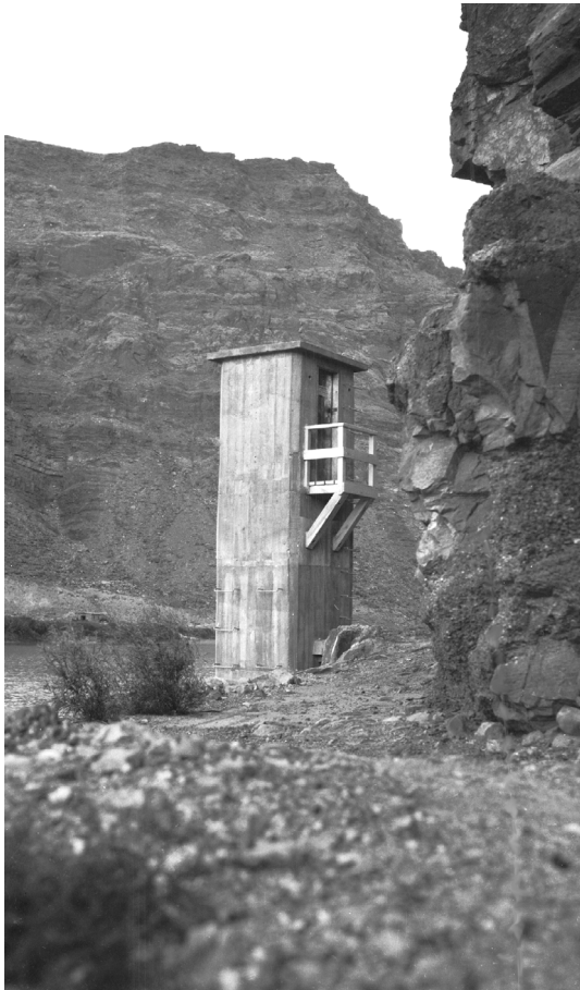
Figure 2. Lees Ferry Gage. (A) View from the right bank downstream from the Number 1 Gage. Photograph taken by G.C. Stevens of the U.S. Geological Survey at 9:00 a.m. on September 21, 1923, when the stage was 11.05 feet and the discharge was 27,000 cubic feet per second. Source of this and the photographs in figs. 2B–3D, and 16B: 1921–37 Surface Water Records File, Colorado River at Lees Ferry, Arizona, file stored at the Federal Records Center in Laguna Niguel, California, in Accession No. 57-78-0006, Box 2 of 2, Location No. MB053635. (B) View from the edge of the dugway road downstream. Photograph taken by G.C. Stevens of the U.S. Geological Survey just after sunset on September 22, 1923.
