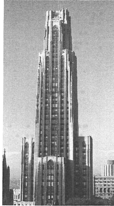
Bellefield Avenue Side (facing NE)
