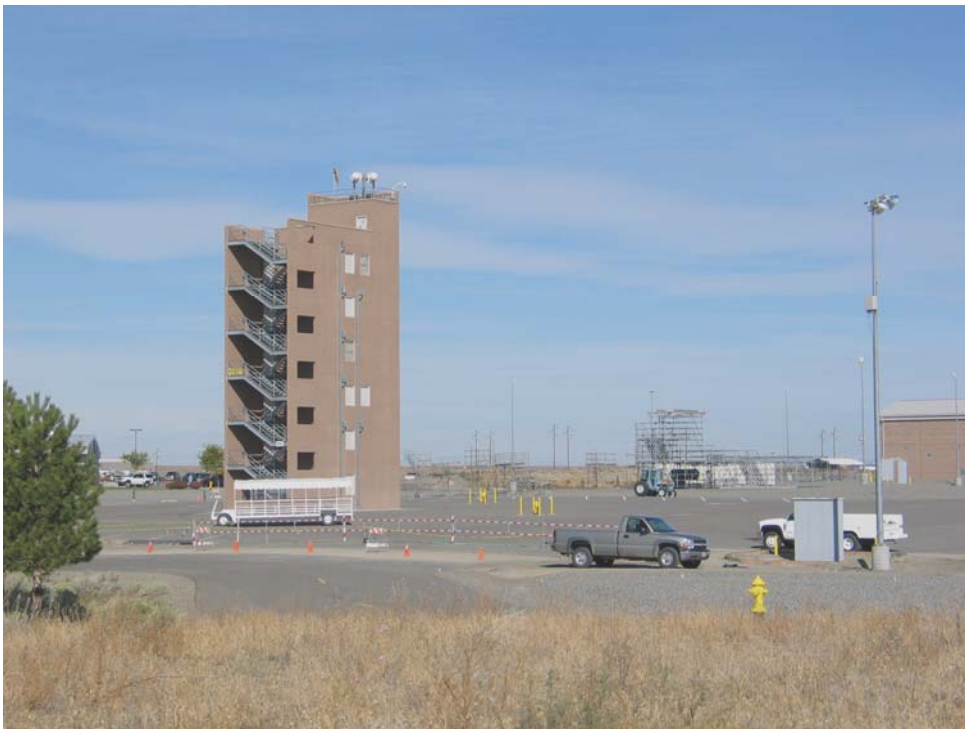
View of part of the HAMMER Training Facility, Hanford Washington
