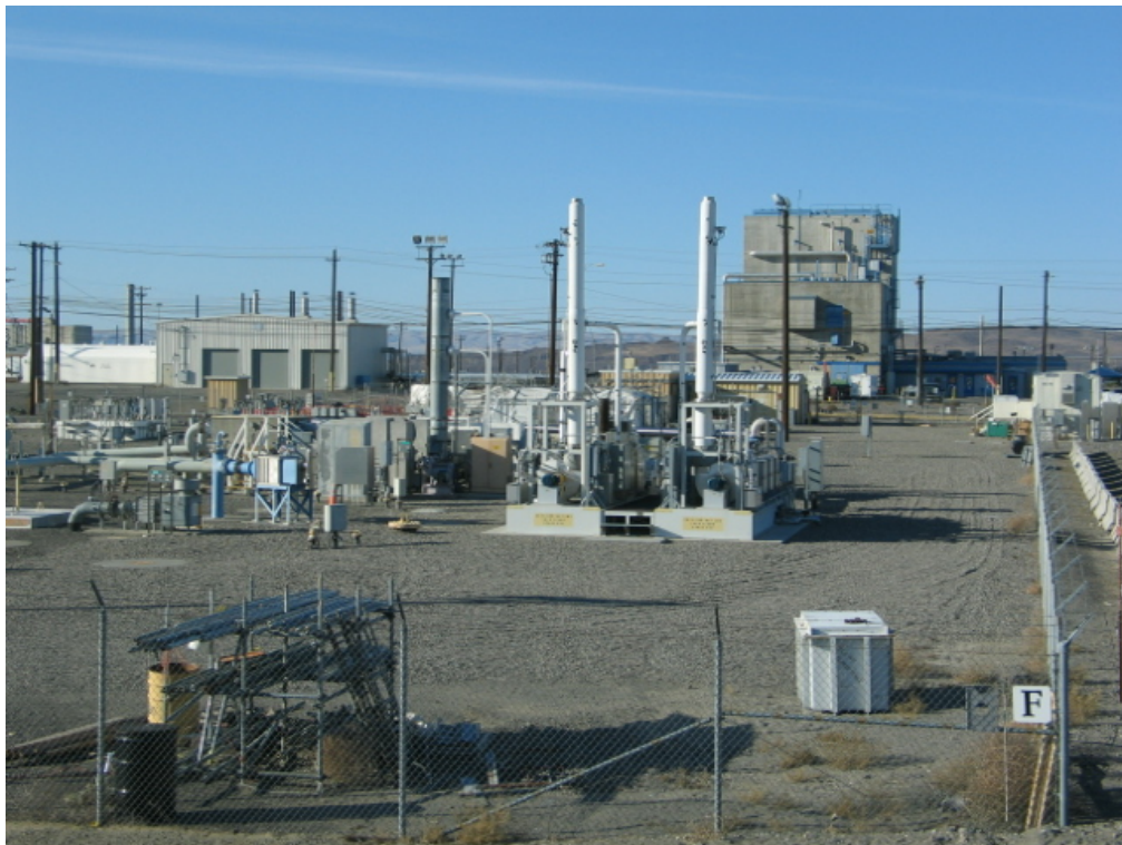
Nuclear Waste Tank Farm, Hanford , Washington
