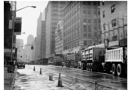
Fig. 3. Trucks on Chambers Street waiting to pick up debris from World Trade Center during the first week in October, 2001. Note that the streets surrounding the WTC were kept continuously wet to suppress the dust.
