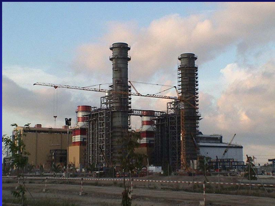
750-MW IPP Ca Mau Gas Combined Cycle Power Plant 1 with Siemens Turbines developed Petrovietnam with USD 436 million in investment Commercial Operation: October 2007
