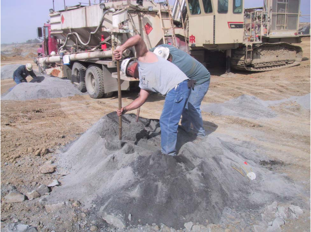
Figure 16 - Stemming the loaded blast hole
