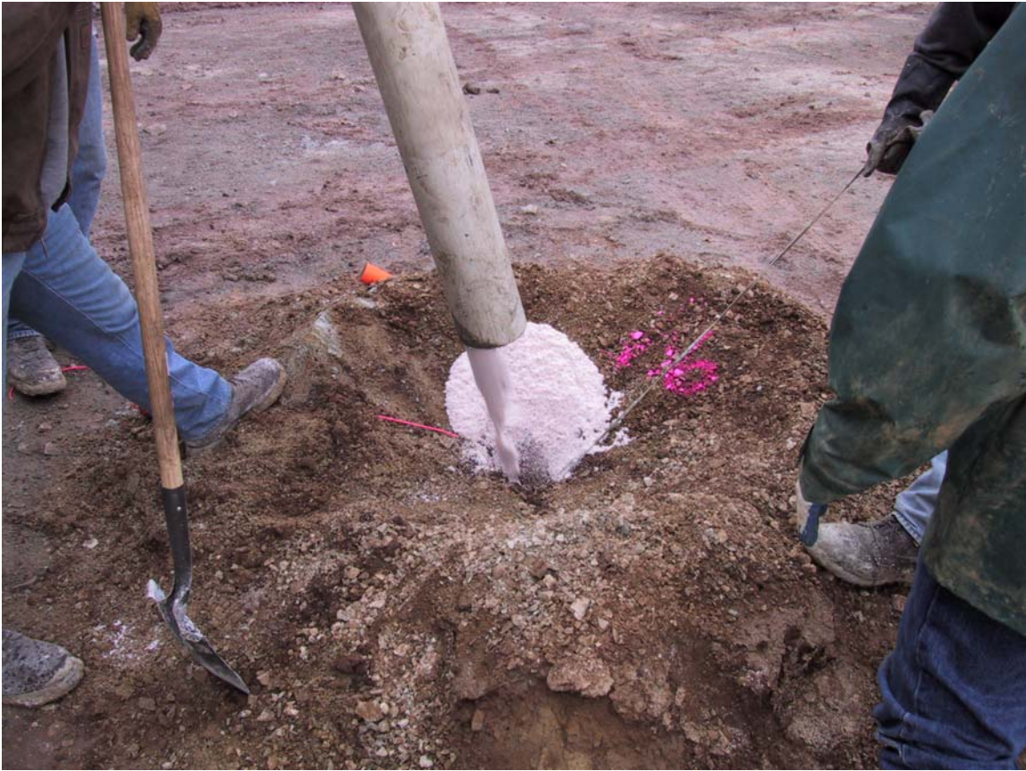
Figure 9 - Loading ANFO into a blast hole primed with a booster and Daveytronic® electronic
