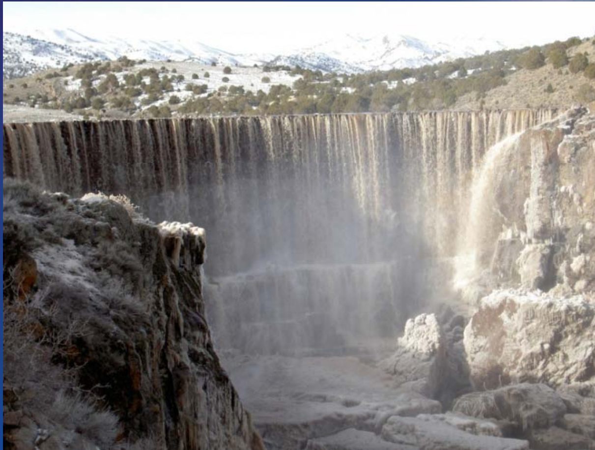
Lower Enterprise Dam - January 13, 2005
