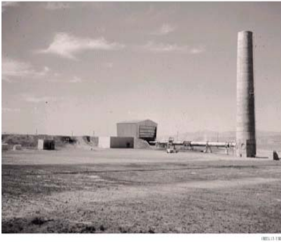
Figure 2-4 150-foot Exhaust Stack
