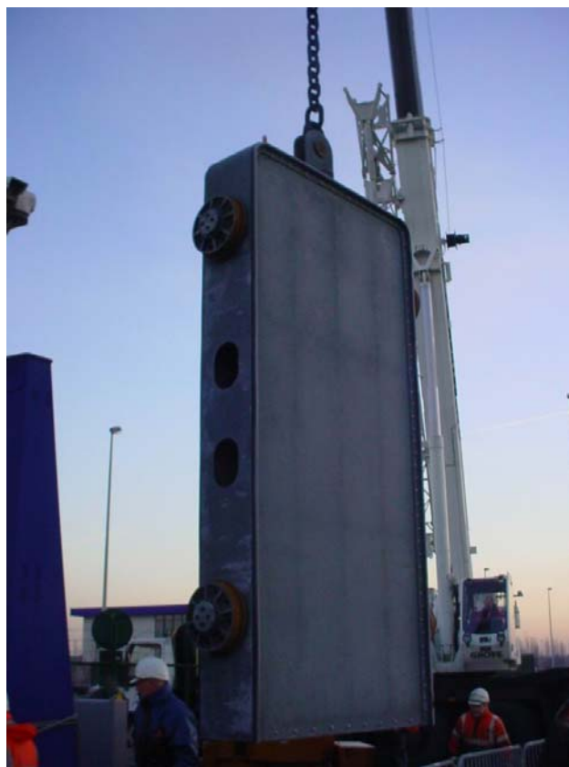
General view of culvert gate
