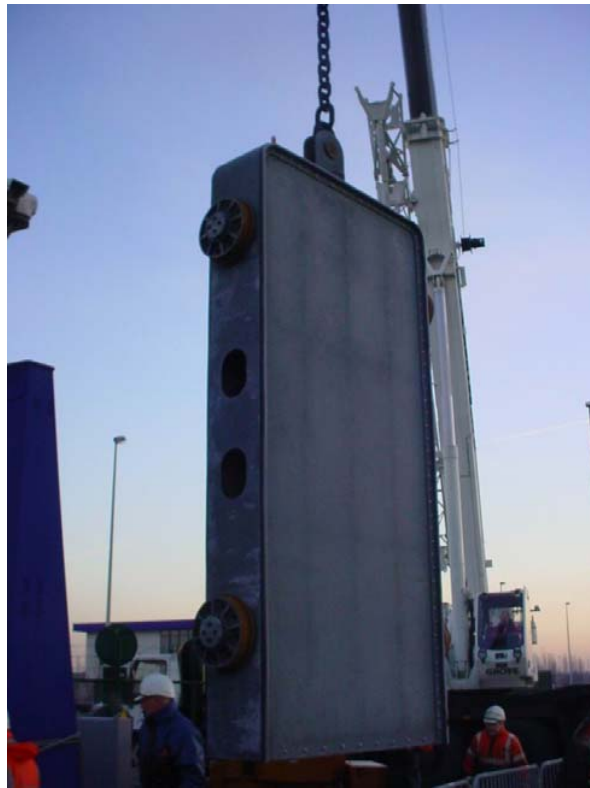
General view of culvert gate
