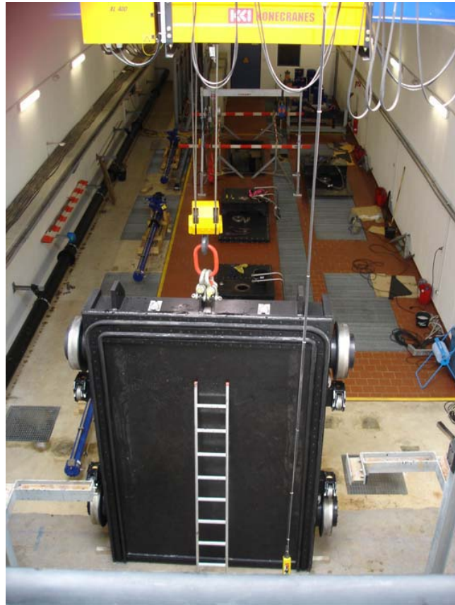
GATES OF WSB OF THE MAGDEBOURG (ROTHENSEE) LOCK SYSTEM
