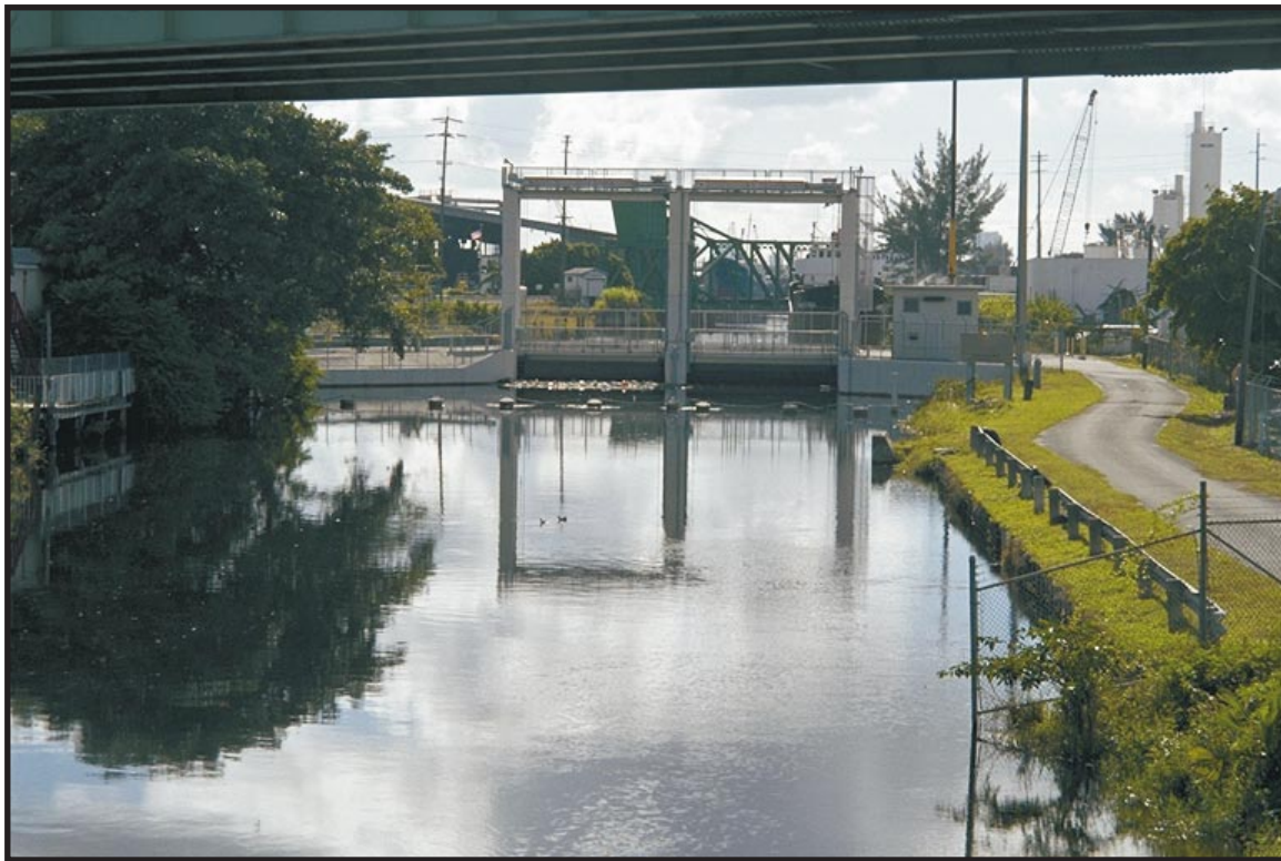
Figure 4. Structure S-26 at the Miami Canal station.
