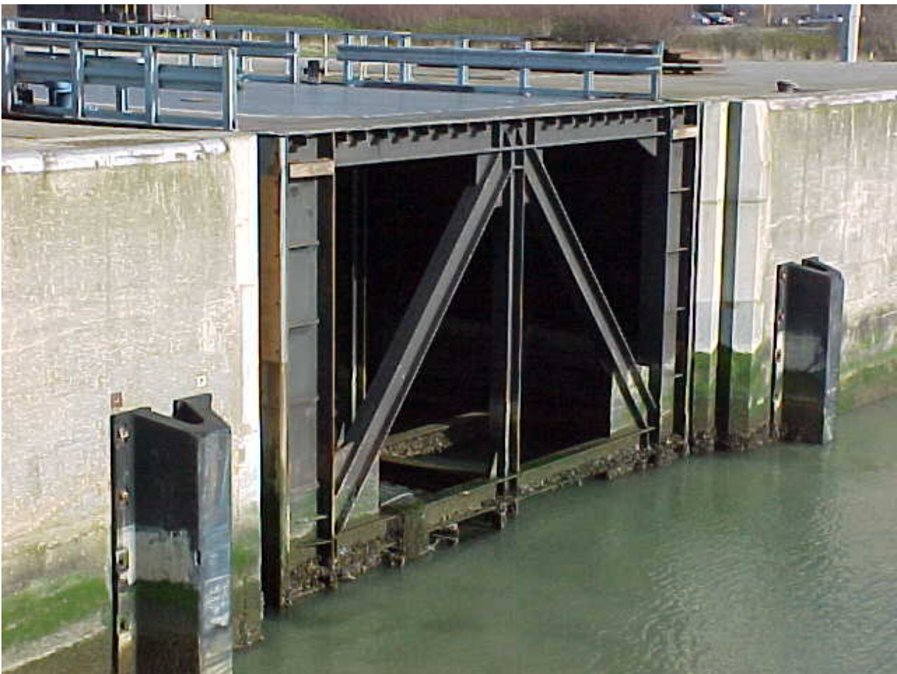
Picture of a rolling gate in its recess in the P. Vandamme lock in Zeebruges – Belgium
