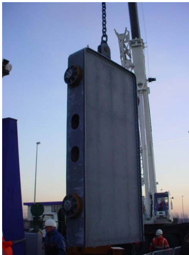
General view of culvert gate
