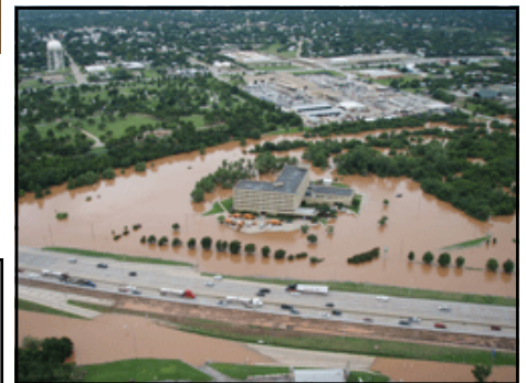
As the river swelled, flood waters surrounded the Holiday Inn in Wichita Falls off Interstate 44. Photo © 2007 Wichita Falls Public Information Office.
