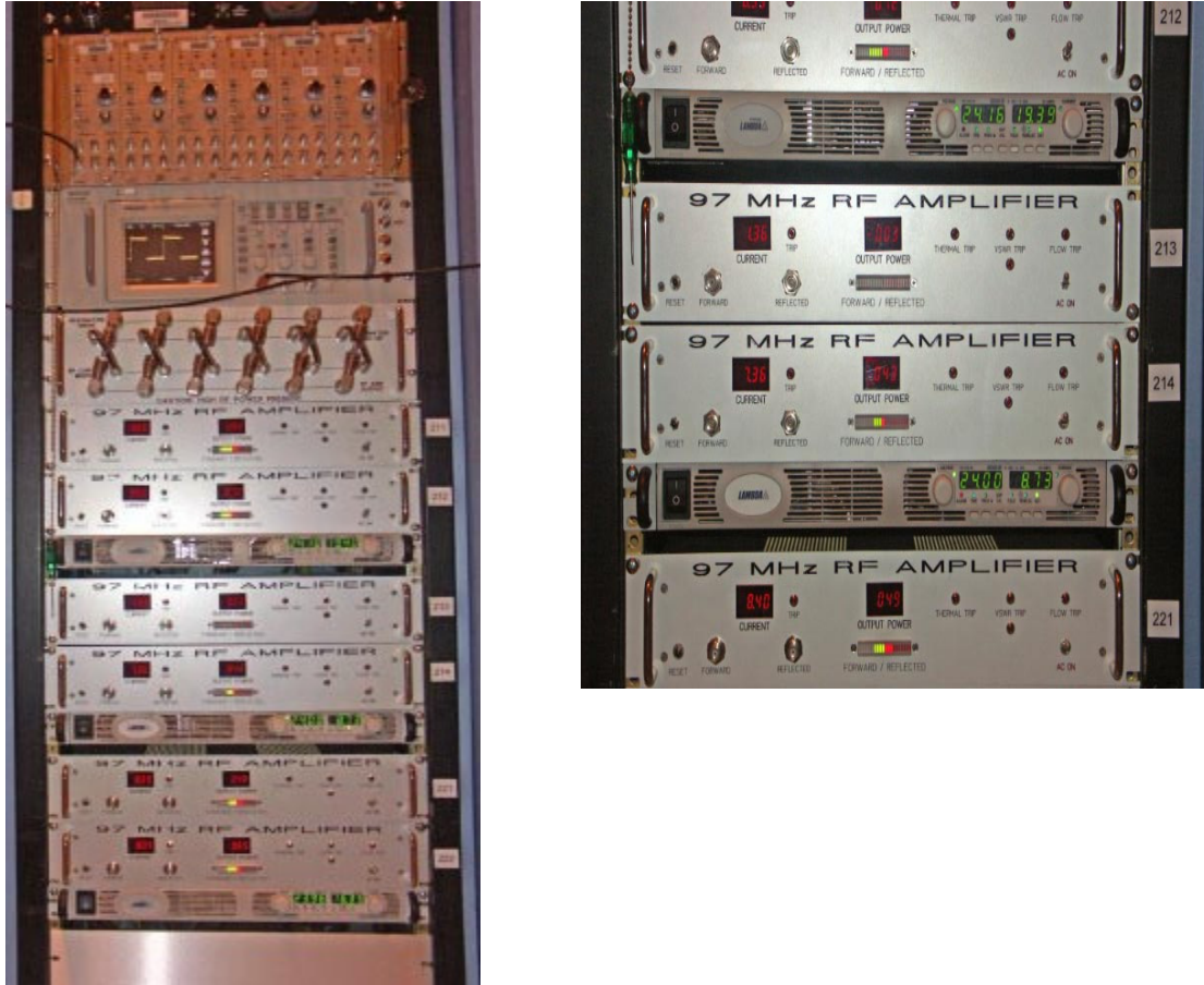
Fig. II-5. A view of the first modified booster rack.
