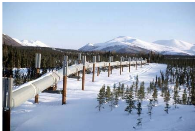
The TAPS includes both buried pipe and pipe supported on steel structure above ground, depending on local soil and geologic conditions.
