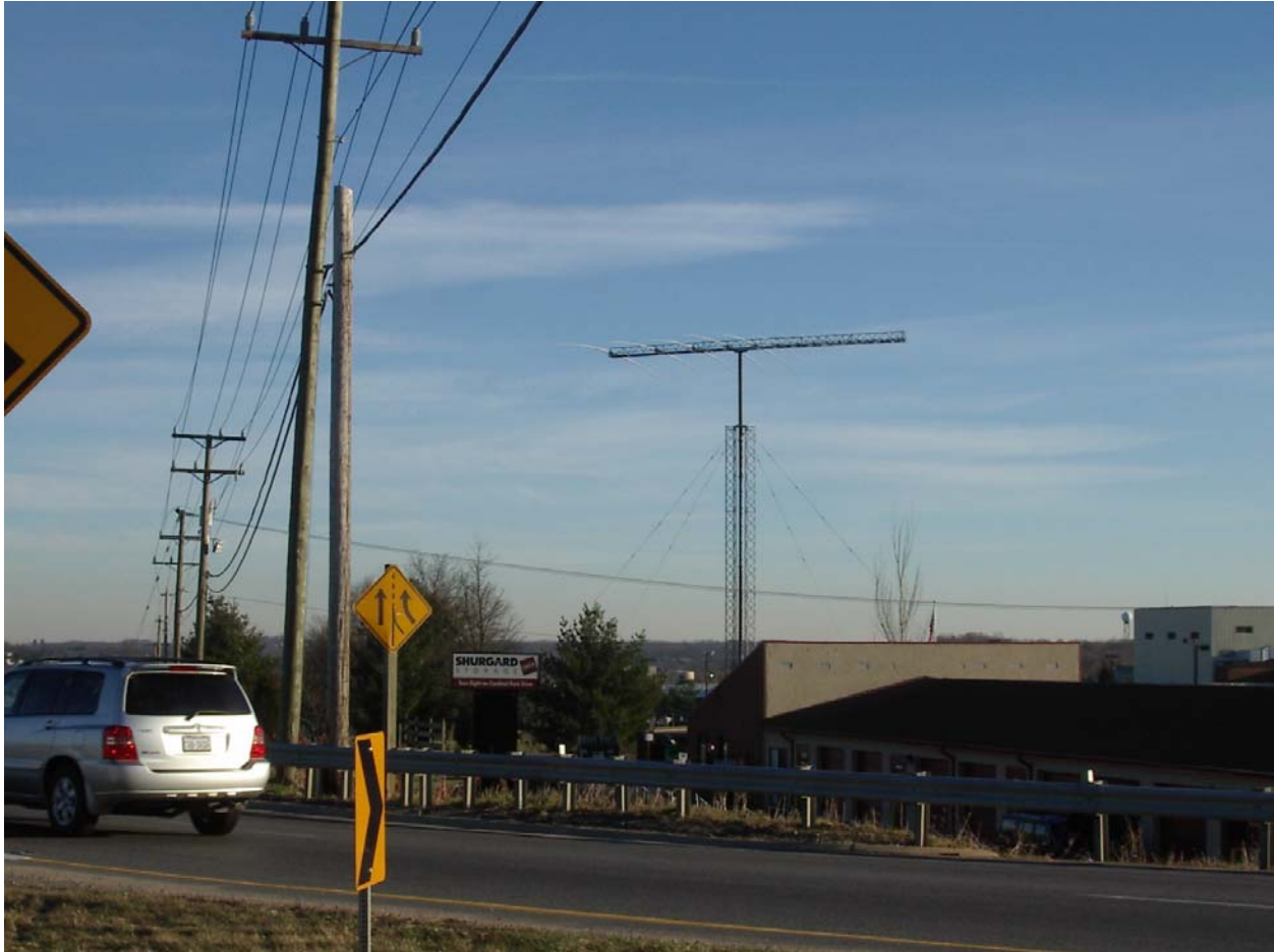
Figure C-1: An Example of a Federal Government Radio Antenna near Power Lines.
