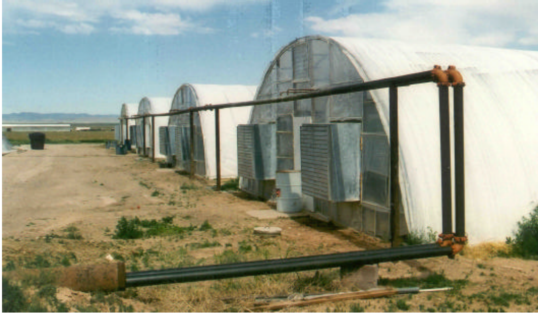
Castlevalley greenhouses showing geothermal water supply lines.
