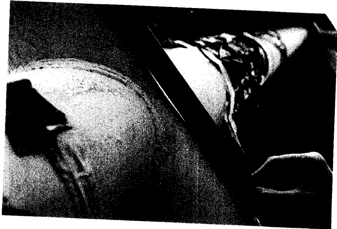
Figure 2.8 Node 42 - Scan 9 - initial signs of chord ovalisation
