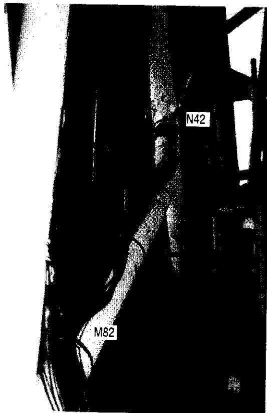
Figure 4.15 Brace 82 buckled and Node 42 distorted at Scan 45
