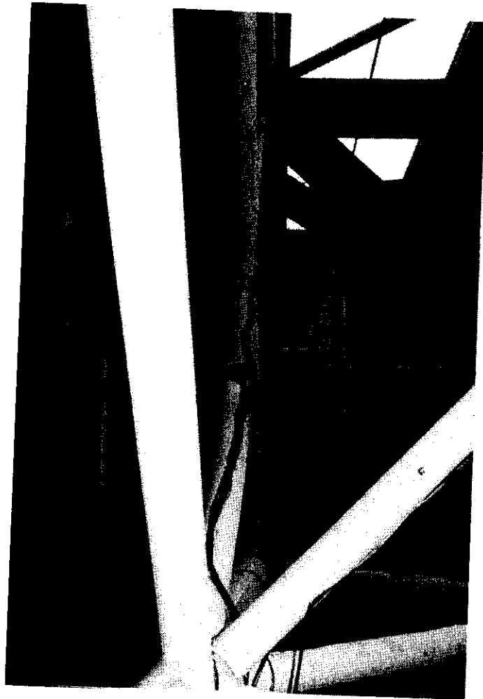
Figure 2.12(a) Brace 78 - Scan 39 - out-of-plane buckling view along Frames A/E leg from Level 2 to Level 3
