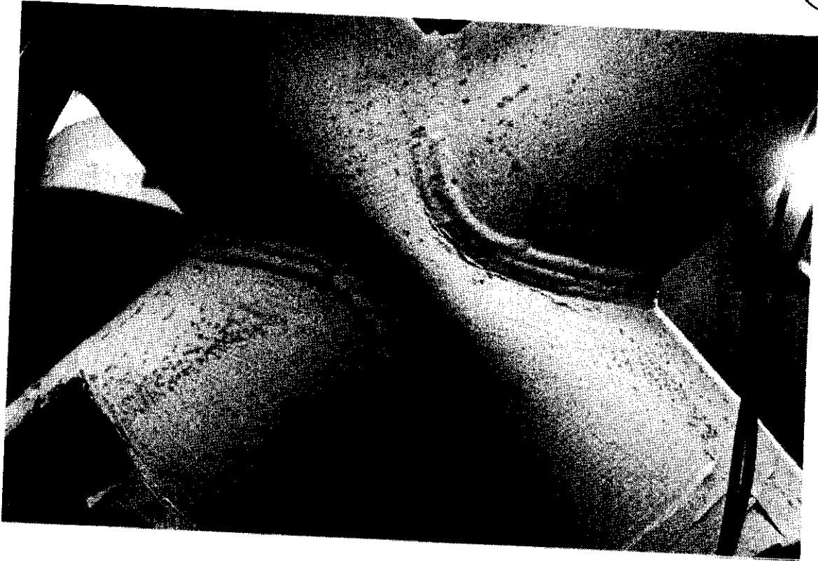
Figure 2.10 Node 42 - Scan 16 - chord deformation just beyond initial peak in capacity
