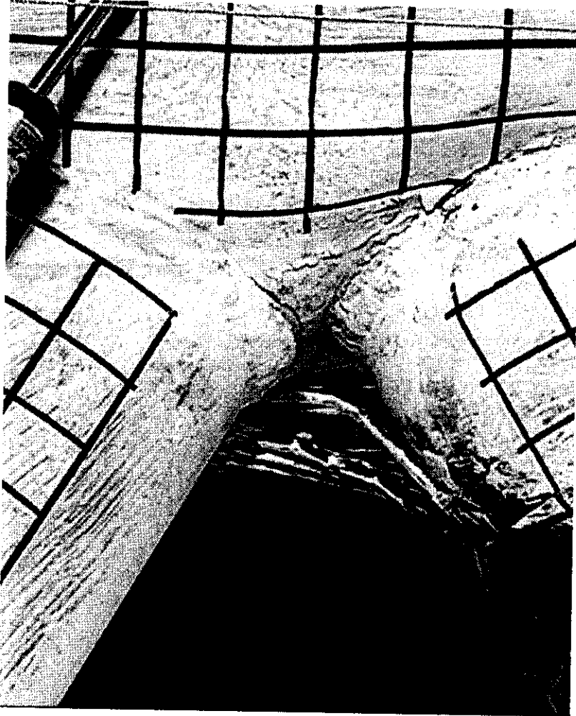
Figure 2.11 Through thickness cracking in gap region of Node 38 at Scan 21
