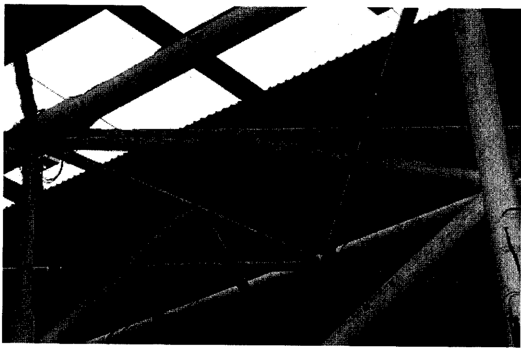
Figure 4.7 Brace 72 - buckled
