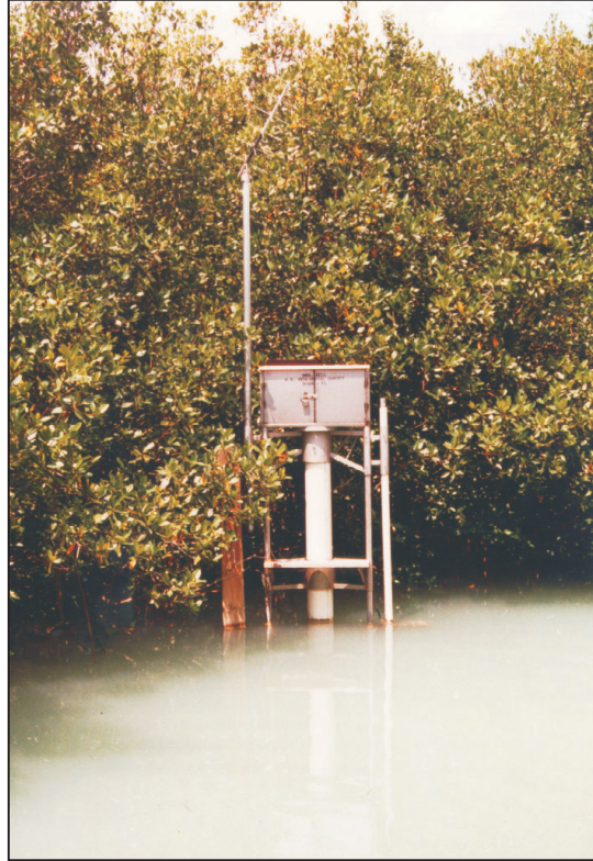
MUD CREEK MONITORING STATION
