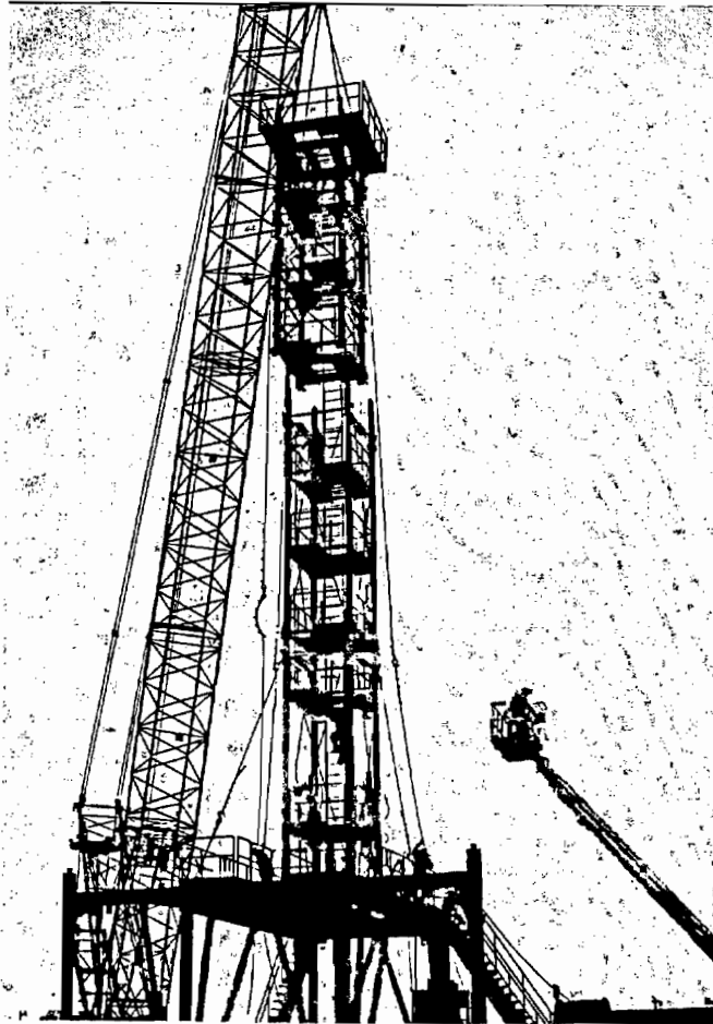
Figure 12-10. Field Erection of Drilling Structure (Frishmuth et al., 1996)
