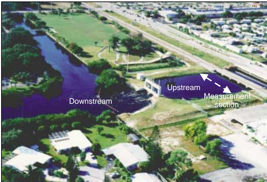
Figure 16. Location of structure 37A.
