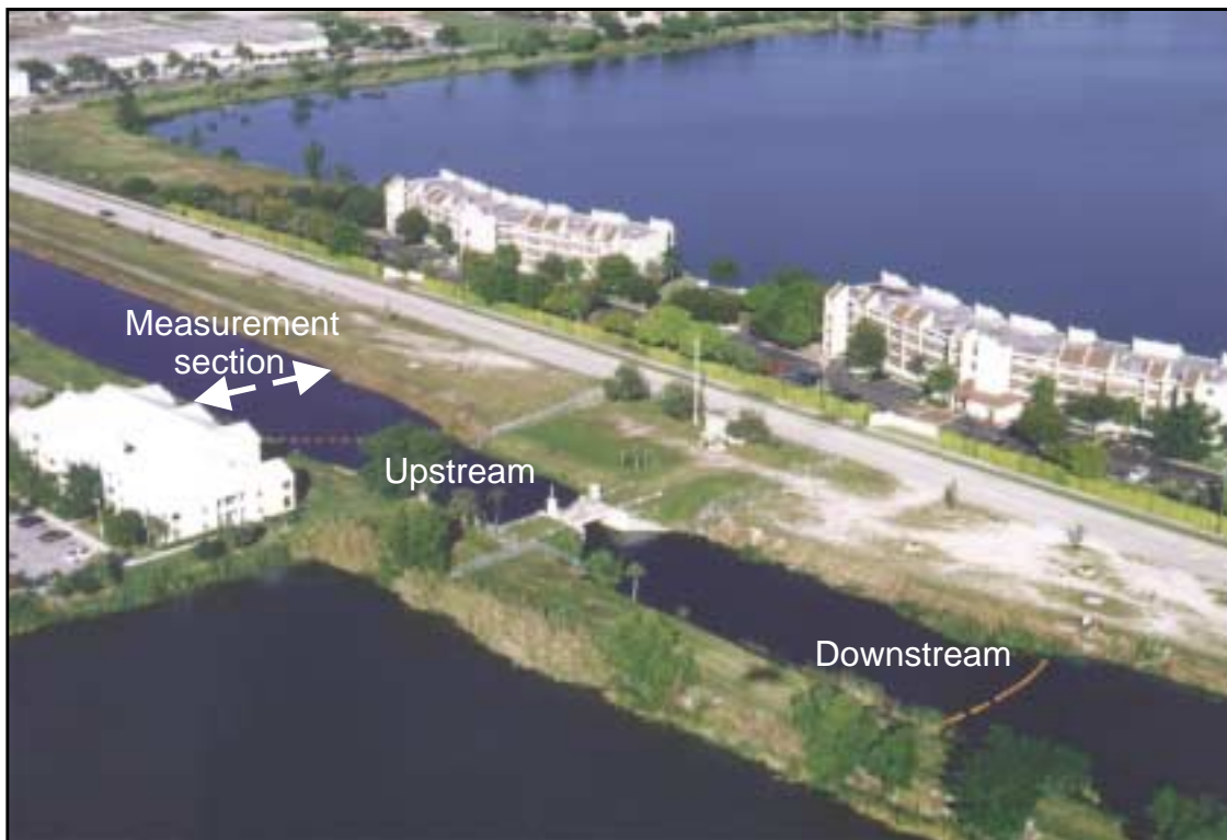
Figure 18. Location of structure S-36.
