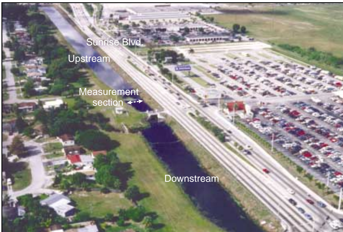
Figure 20. Location of structure S-33.
