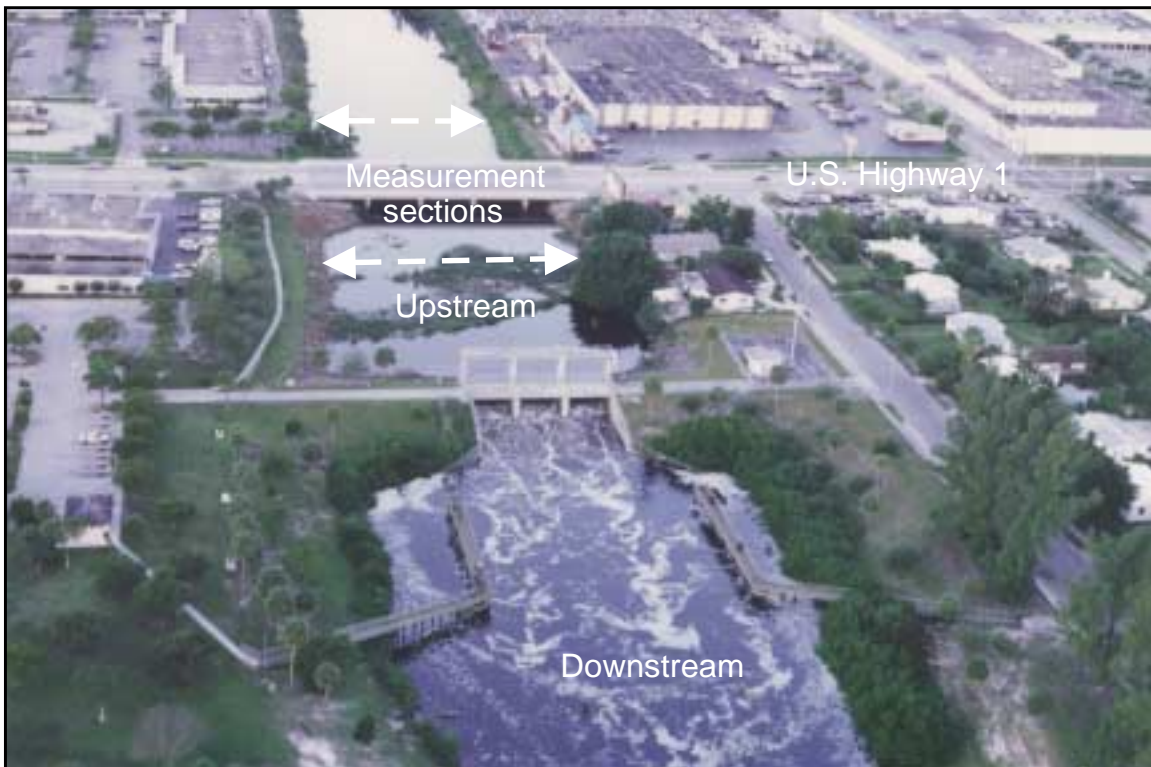
Figure 6. Location of structure S-155.
