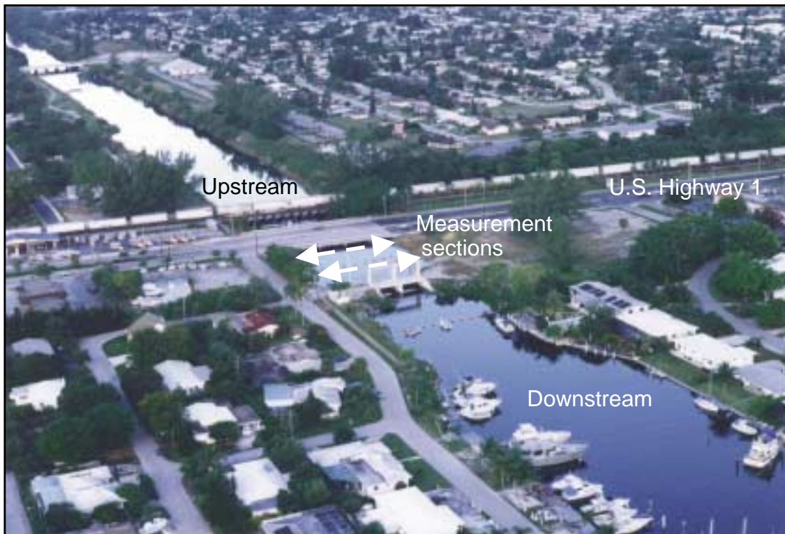
Figure 8. Location of structure S-41.
