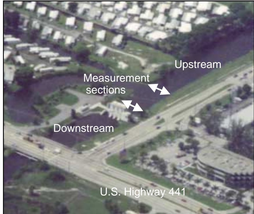
Figure 24. Aerial photograph showing location of structure S-13.
