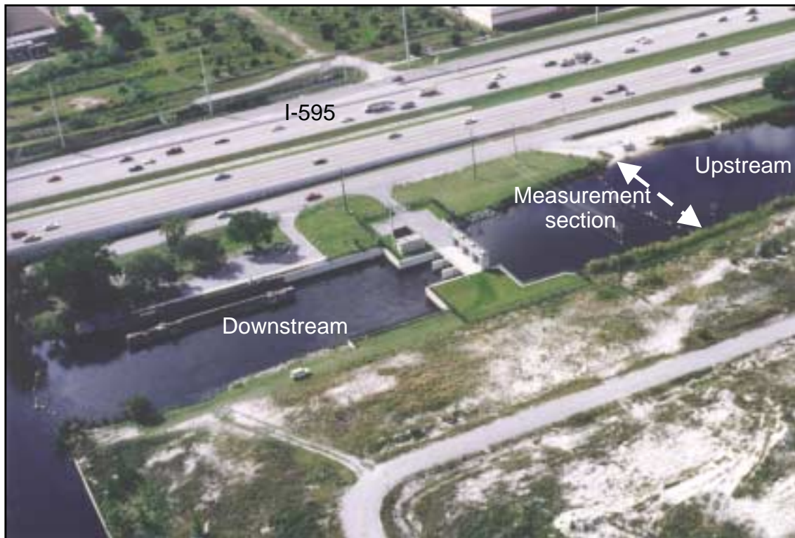
Figure 22. Location of structure G-54.
