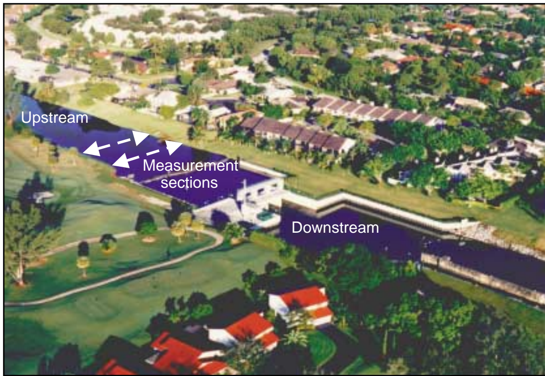
Figure 12. Location of structure G-56.
