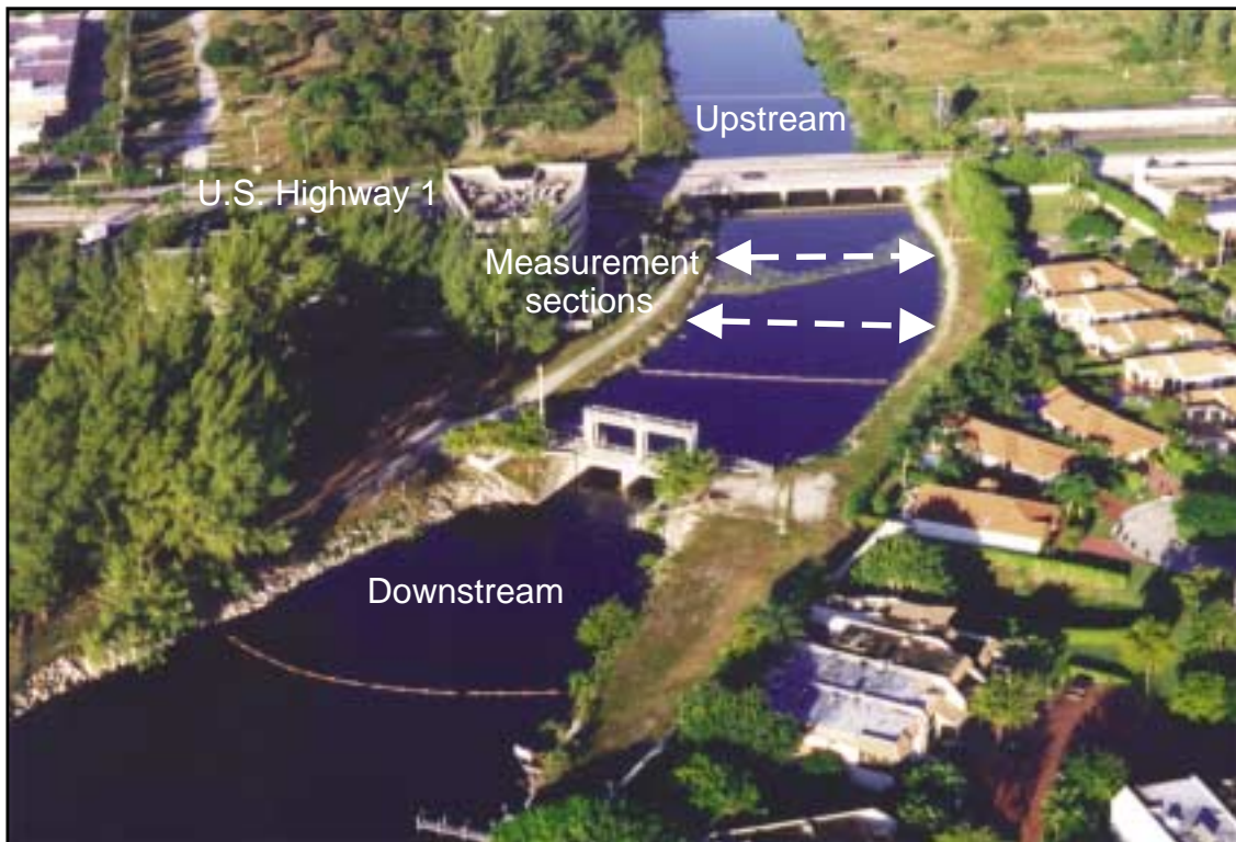
Figure 10. Location of structure S-40.
