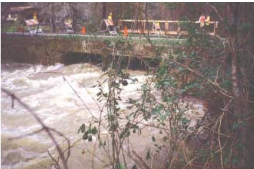
Lafayette Creek flood water on the downstream side of Miccosukee Road
