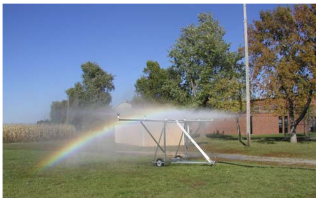
Specially designed spray irrigation equipment treating contaminated groundwater in Nebraska.
