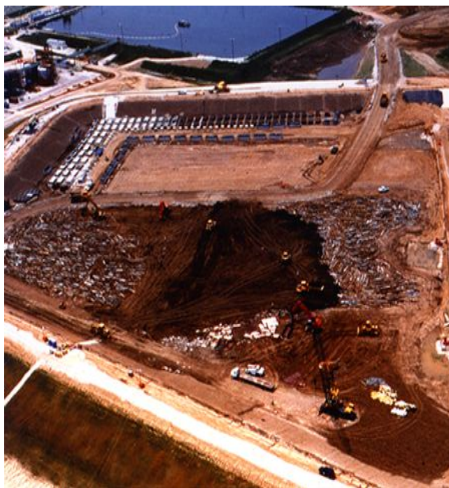
Disposal cell development
