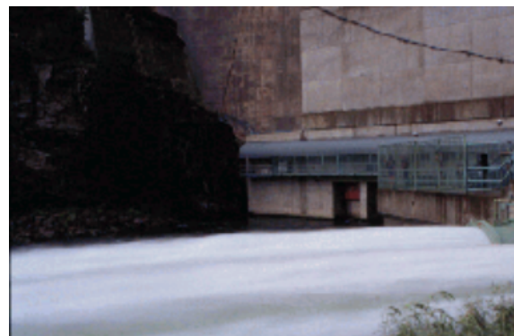
Bypass release at Flaming Gorge Dam in June 1997
