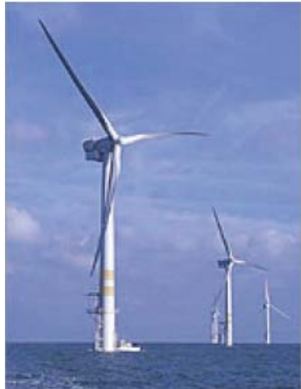
Wind Energy Facility Operating off the Coast of Ireland (Source: DOE)
