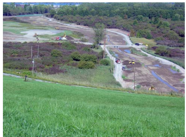
Site restoration of Rattlesnake Creek after remediation
