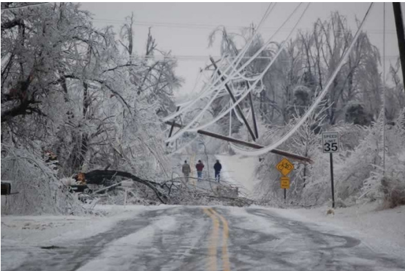
An example of the extreme ice damage that occurred with the January 26-27 ice storm in northwest Arkansas.
