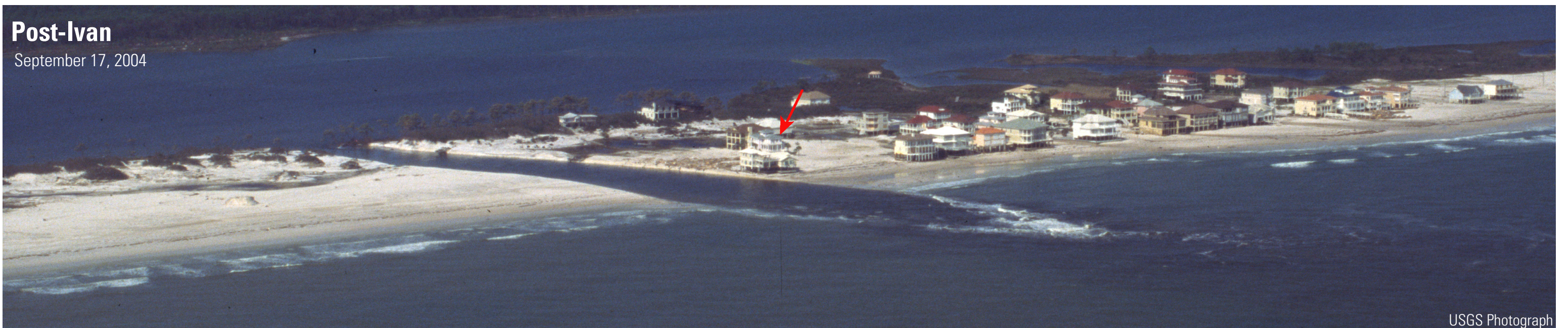
Figure 3. Pine Beach, Alabama. Top and Center: Topography/bathymetry measured with lidar before and after the impact of Hurricane Ivan showing a new breach that severed the island. (Note the new houses that were built between the surveys. Houses appear in the topography as rectangular mounds. Their warmer colors indicate higher elevations.) Bottom image: A USGS aerial photograph shows the new breach following landfall. (Arrows in all images point to the same features.)
