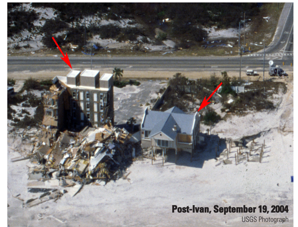
Figure 2. Orange Beach, Alabama. USGS aerial photographs taken before and after the landfall of Hurricane Ivan show the failure of a five-story condominium tower. The only parts of the structure that remain standing after Hurricane Ivan are the elevator and stairwell shafts. Airborne laser mapping data showed that the sand dune on which this building was constructed was subjected to about 3 m of vertical erosion during the storm. (Arrows in all images point to the same feature.)
