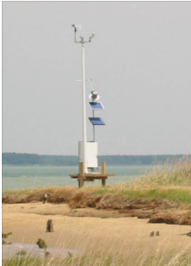
Figure 2. Barren Island water level station featuring GOES antenna, solar panels, barometer, and wind sensor.
