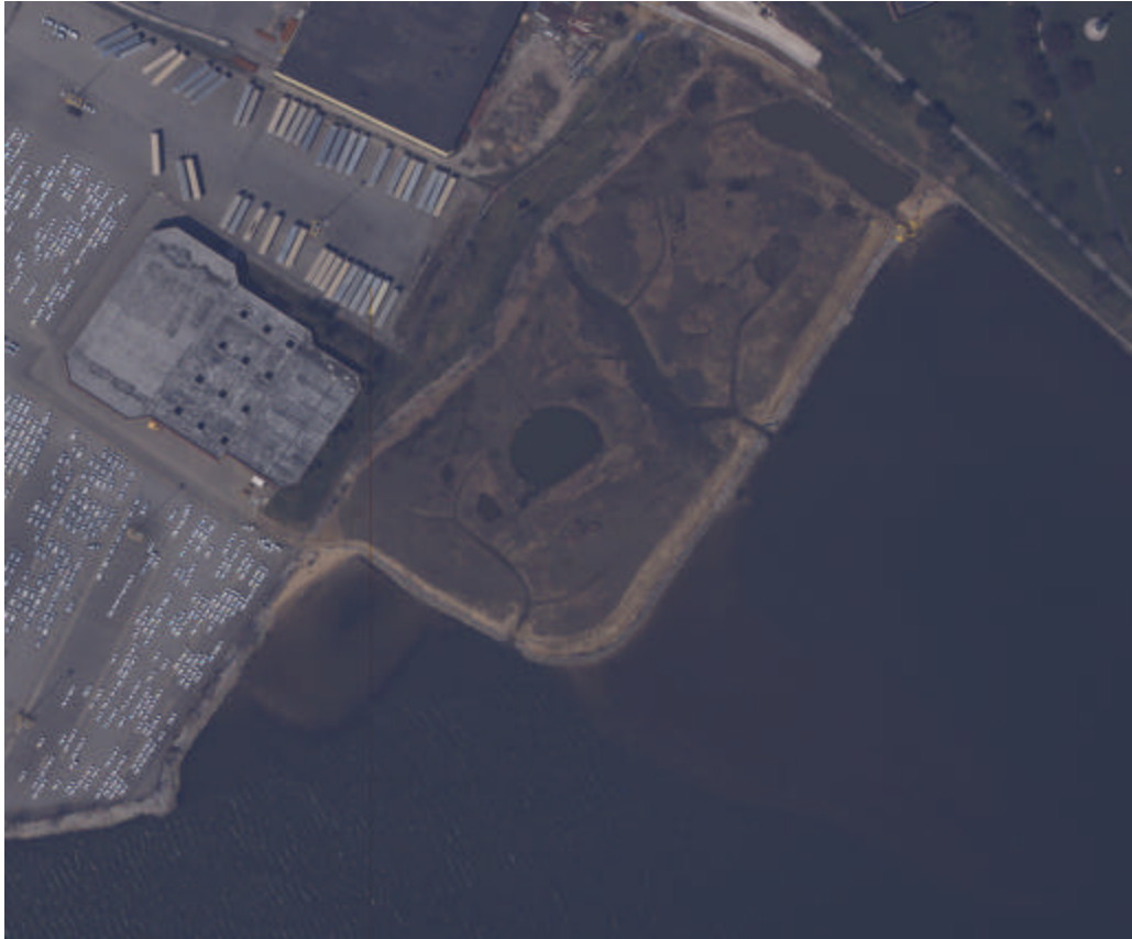
Figure 20. Aerial photographic image of the wetlands after completion of construction.
