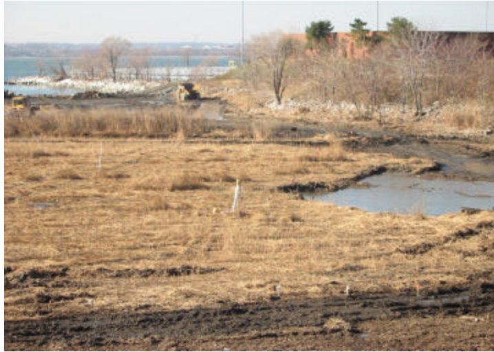
Figure 11. Photograph showing the use of the leveling transit to control the marsh surface.
