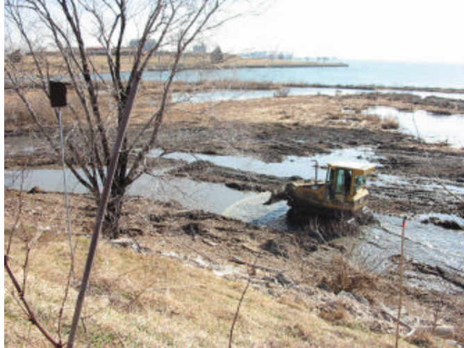
Figure 13. Photograph showing the grading of the surface of the wetlands.
