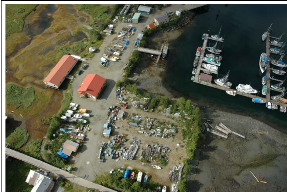
All buildings and structures are mapped as wharves (Form "Aw"); other Forms include marina ("Am"), breakwater ("Ab"), and debris classified as fill and tailings ("At")
