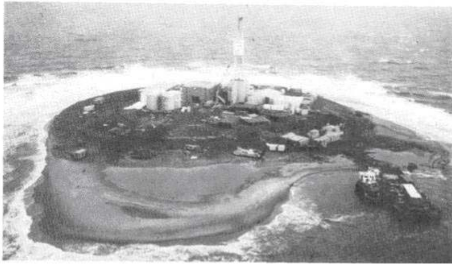
Figure 3-69: Imperial Oil's Arnak L-30 September 1976 Showing Wave Action on the Sacrificial Beach Island Design (from Croasdale and Marcellus, 1977)
