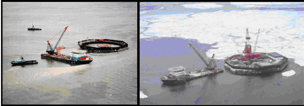
Figure 3-56: Esso's Caisson-Retained Island (CRI)
