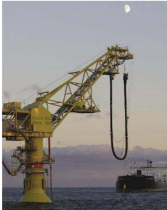
Figure 4-39: The Sakhalin 1 Fixed Tower SPM Sits 61 m above the Seabed (Courtesy of PennWell Publishing, 2007)
