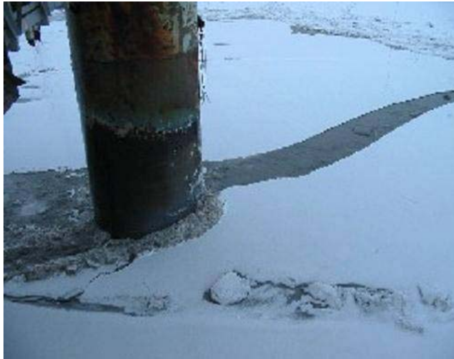
Figure 4-11: Sea Ice Loading a Jacket Leg, Cook Inlet (Courtesy of CIRCAC, 2007)
