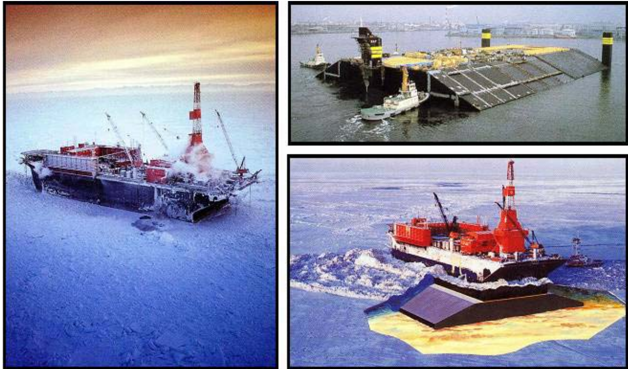
Figure 3-55: SSDC (left), MAT Substructure (Top Right), SSDC/MAT (Bottom Right)
