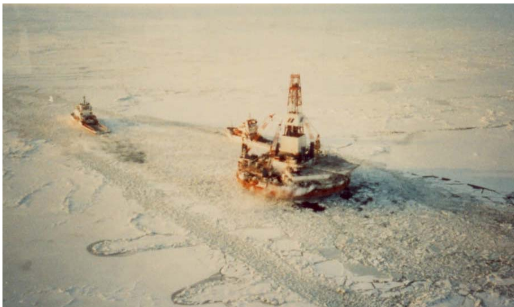
Figure 3-75: The Kulluk - Operations with Icebreaker Support (Courtesy of DC Marine)
