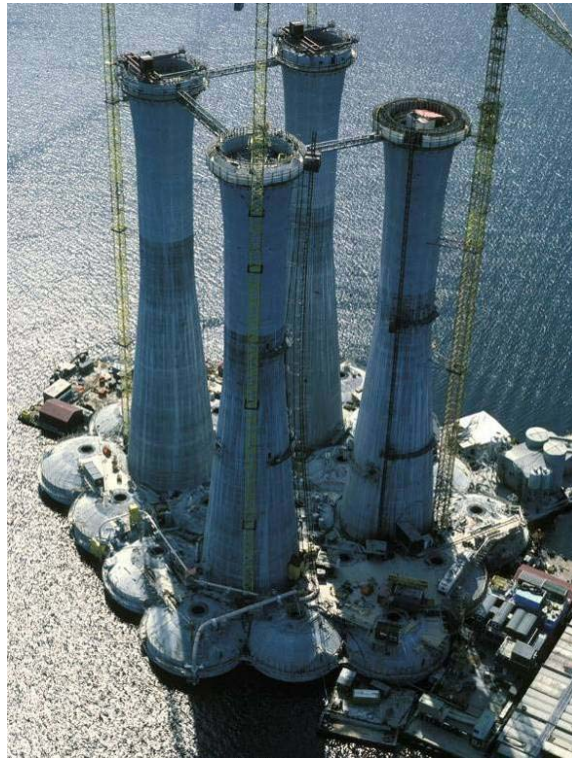
Figure 3-62: Statfjord C under Construction (Statoil ASA, 2007)
