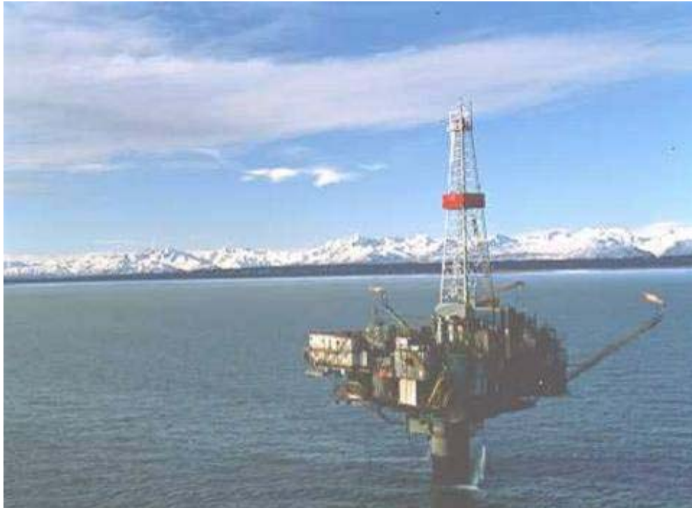
Figure 4-10: Unocal's Monopod Jacket Platform, Cook Inlet (Courtesy of CIRCAC, 2007)
