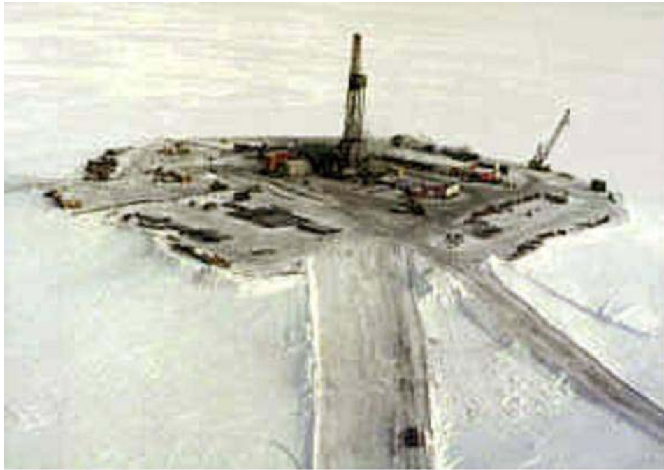
Figure 3-65: Mars Spray Ice Island (C-CORE, 2005)
