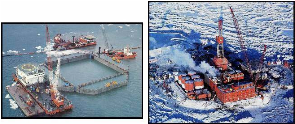
Figure 3-54: Tarsiut Concrete Caissons during Installation and in Service
