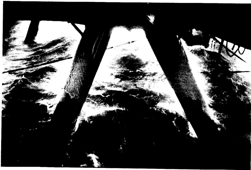
Figure 9. Ice accumulation on diagonal cylindrical trusses under rig (immediately aft of below-deck porthole), which reached a thickness of about 5 in. at bottom, tapering to near zero at underside of main deck. View southwest from below-deck porthole of aft port area (6 January 1983).
