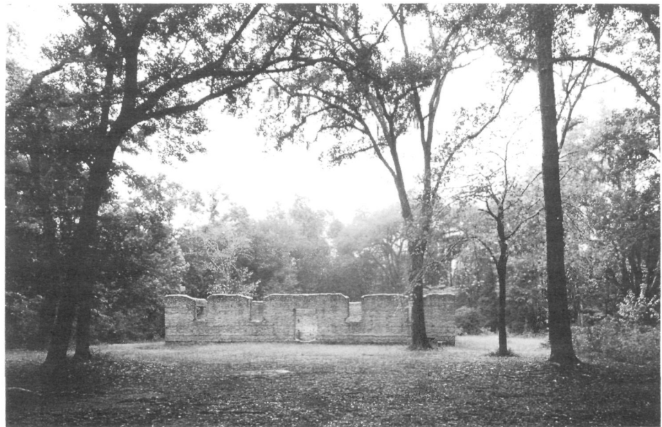
John Houstoun McIntosh Sugarhouse, Camden County, Georgia. The tabby wall ruins of the sugarcane, facing west. (James R. Lockhart)
