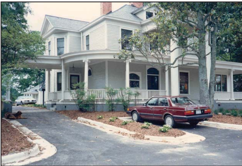
The new parking lot completes the drastic alteration of the setting. The second relocated structure (C2) can be seen through the porte-cochere at left.
