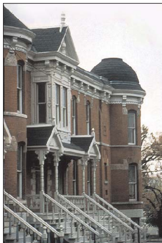
Right: Historic row houses retain their historic character on their primary elevations after rehabilitation.
