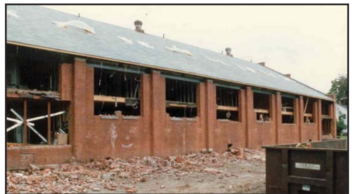
Left: Before rehabilitation the rear elevation of the drill shed, which is highly visible, is distinguished by paired, multi-pane wood windows in the bays. Right: During rehabilitation the historic windows were removed and the openings were enlarged.
