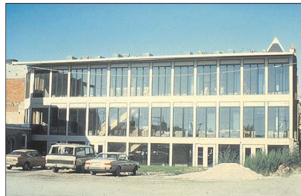
Above: The rear walls of the row houses were covered with a single glass curtain wall that is incompatible with the character of the historic houses as well as the character of the historic district.
