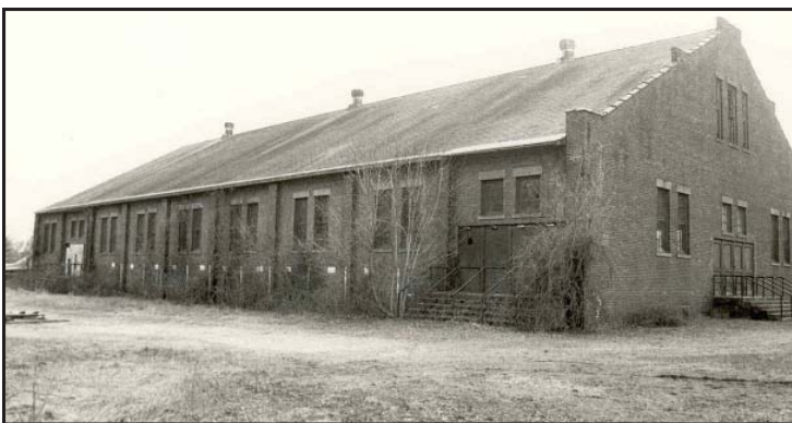
Left: Before rehabilitation the rear elevation of the drill shed, which is highly visible, is distinguished by paired, multi-pane wood windows in the bays. Right: During rehabilitation the historic windows were removed and the openings were enlarged.
