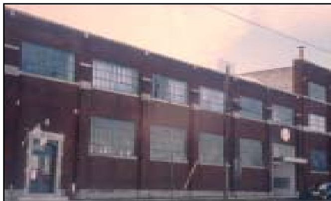
This small manufacturing building had brick walls in the industrial spaces, but several offices on the first floor had finished plaster walls.
