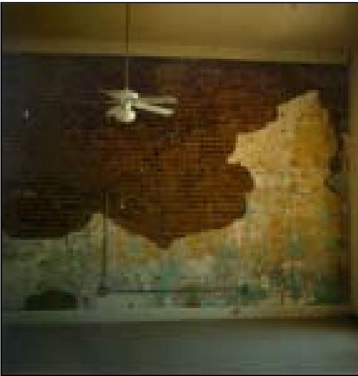
Keeping deteriorated plaster fragments as found without repairing the plaster finish is not an appropriate rehabilitation treatment for most historic building interiors.
