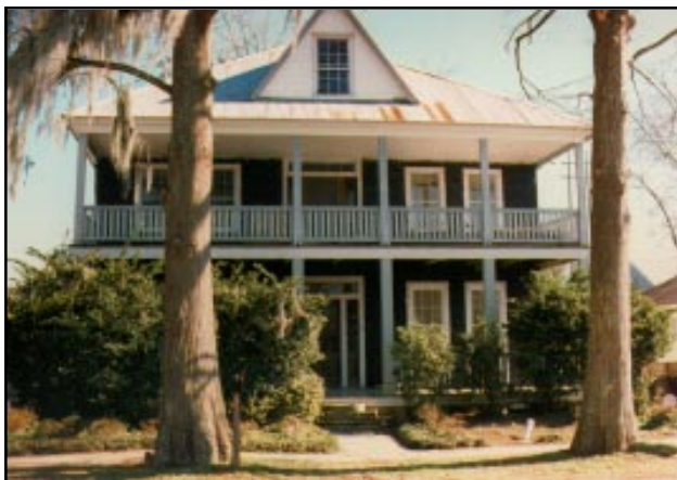
Before rehabilitation - simple historical balustrade.
