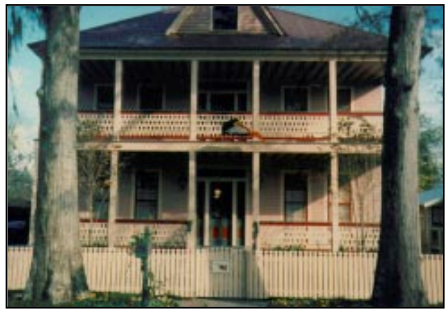
After rehabilitation - inappropriate replacement balustrade.
