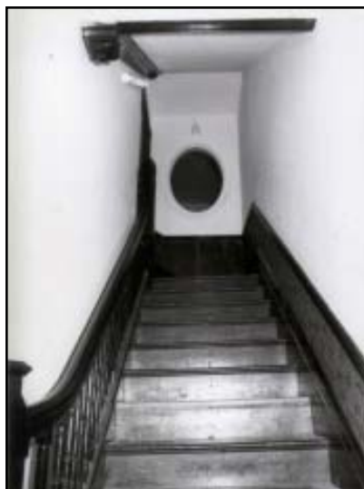
Main hallway, before rehabilitation. The main staircase was enclosed in the 1950s when the house was converted into a five-unit apartment building.
